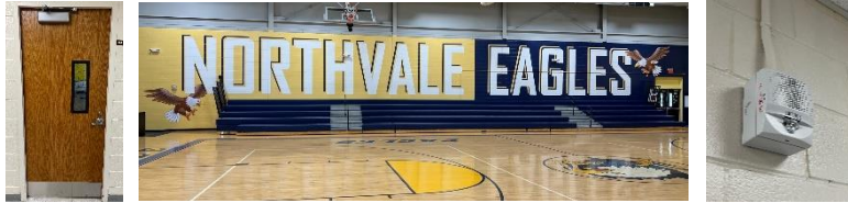
L to R: New Doors, New Wall Graphics, Upgraded Fire Alarm System
